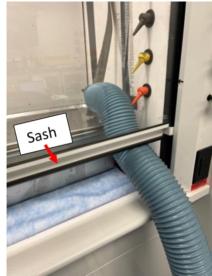
Figure 3. The fume hood safely removes laser cutting exhaust from the room.
